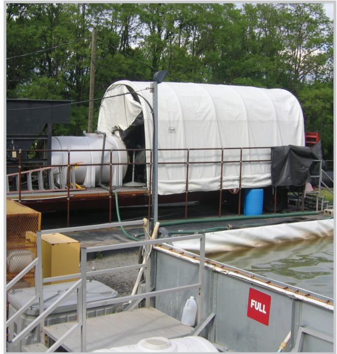
The water treatment system settling tank is in the lower right corner. The ion exchange vessels and activated carbon filter are housed inside the white tent.
